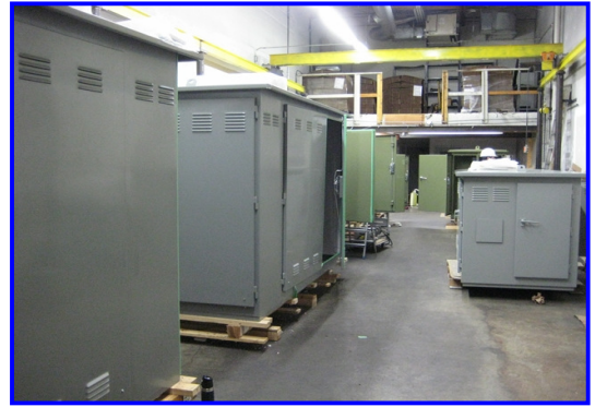
Pump Lift Station
